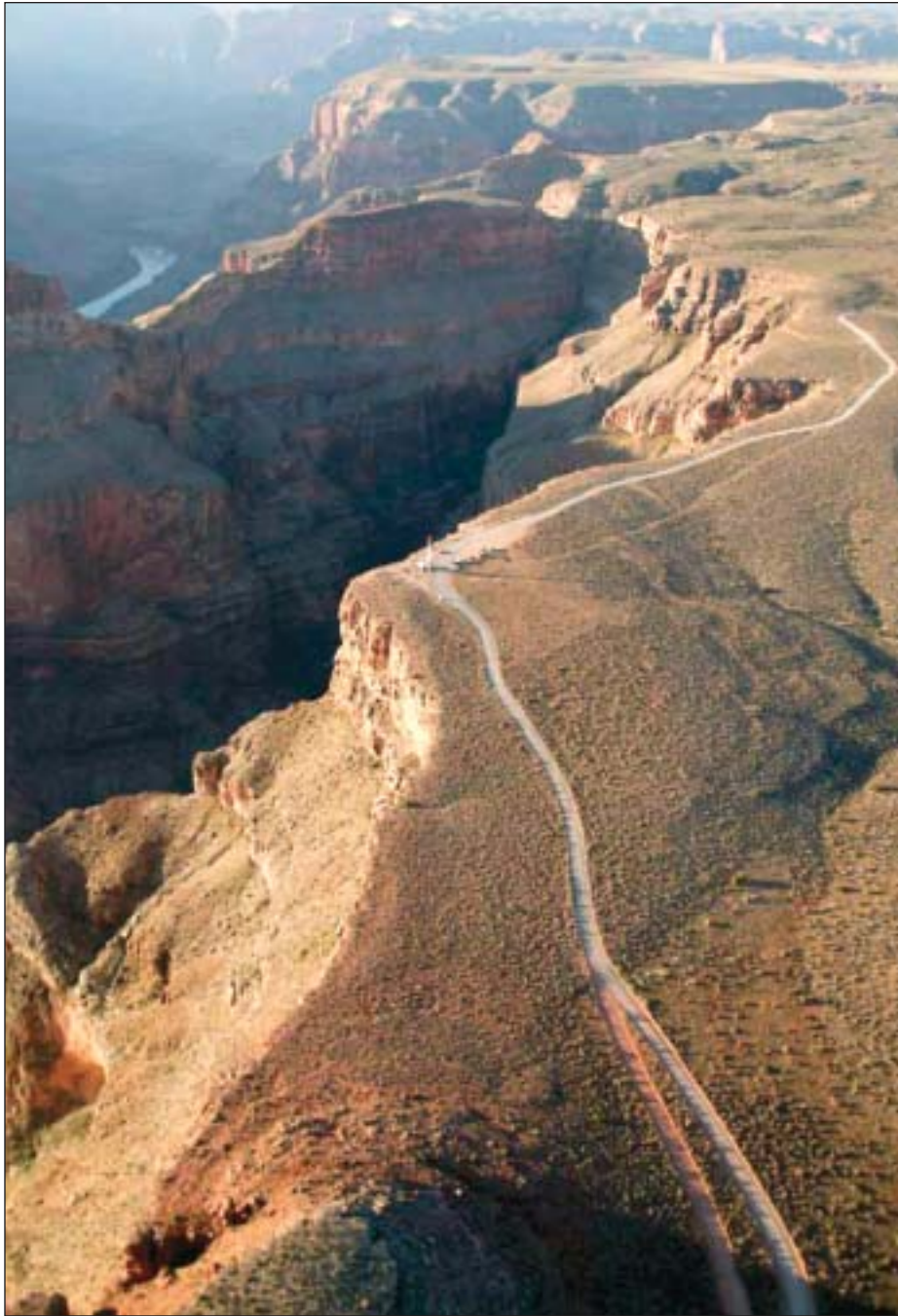
This photo shows the remoteness of the area and the difficulty in bringing in equipment and concrete.
