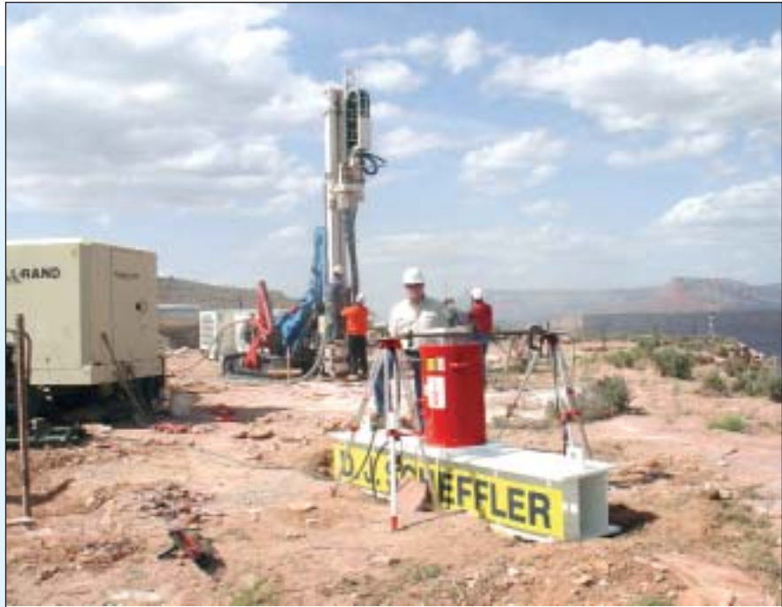
Equipment used to test the micropiles to over 500% of design adhesion.
