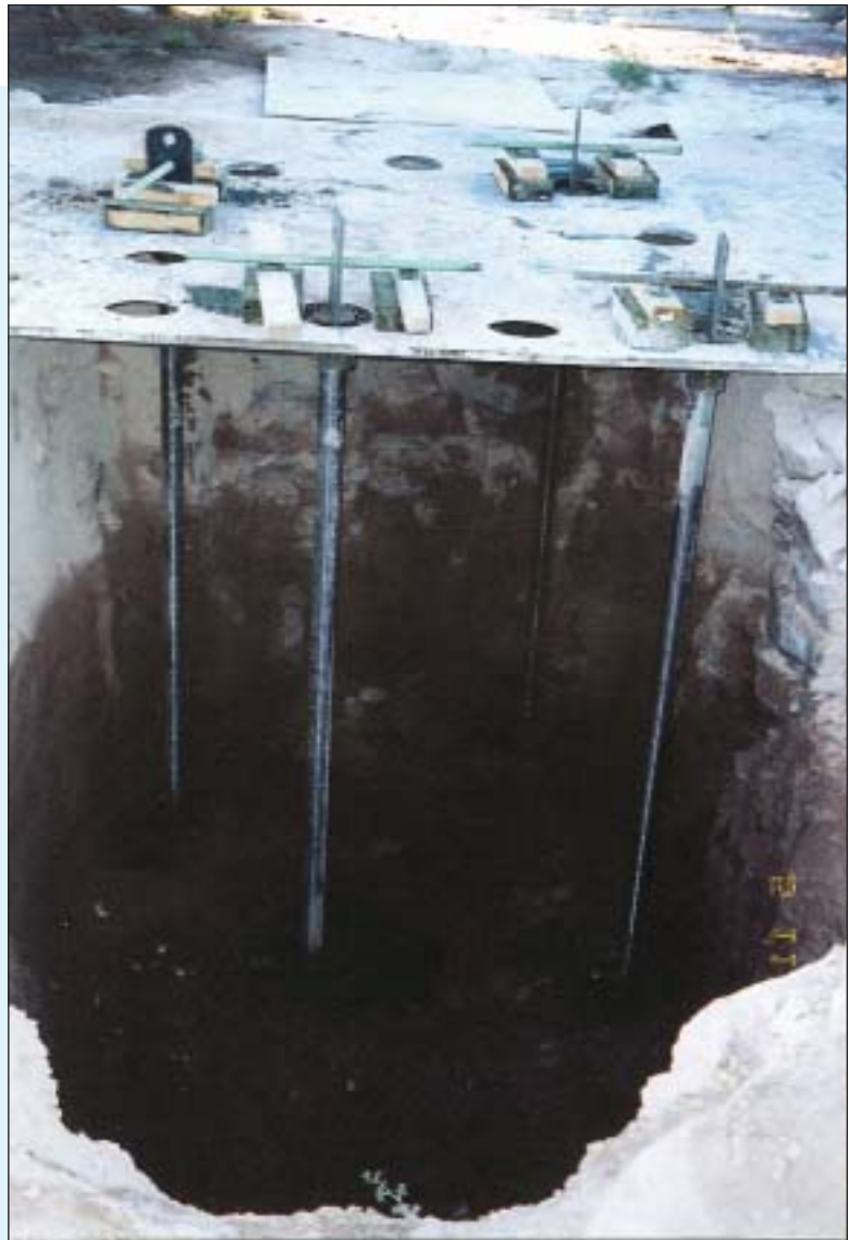
View of excavated pile cap with some of the vertical micropiles installed through steel plate template.
